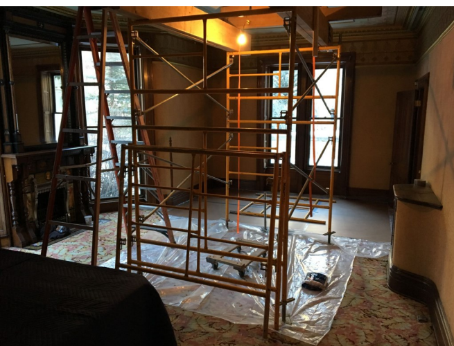
Scaffolding holding up parlor ceiling
